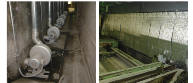
Air distribution fan (left) and heat retention curtain (right) newly installed to stabilize temperature inside curing chamber
